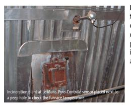
**Pyro-Contrôle,** the expert in temperature sensors, proposes types of protective sheaths which have demonstrated exceptional performance in domestic and industrial waste incineration applications.
